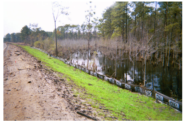
Silt fencing and seeding of side slopes
