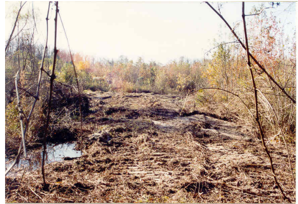
Temporary haul road through wetland
