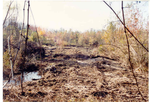
Temporary haul road through wetland
