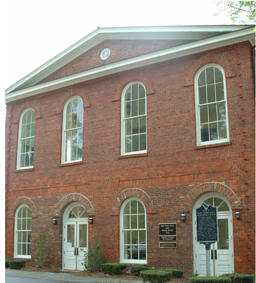
Marion Old Town Hall and Opera House 1892
